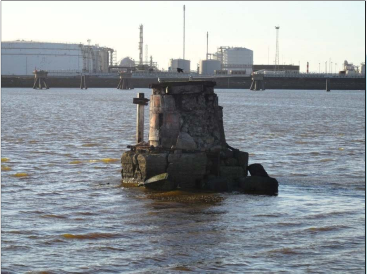
Plate 3: Dolphin Mooring Bollard believed to be located at the recorded location of the Seventh Buoy Light (63) within the proposed scheme footprint for the harbour facility.
